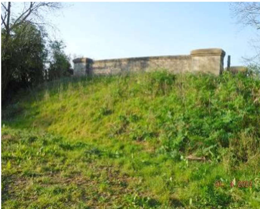
Figure 2.1 – Southern Bridge Elevation Post works
