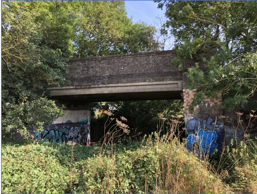
Figure 1.2 - View of the southern former elevation of the bridge structure
