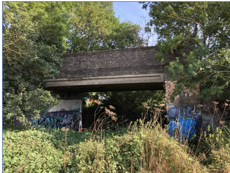
Image 1 - View of south elevation access below structure
