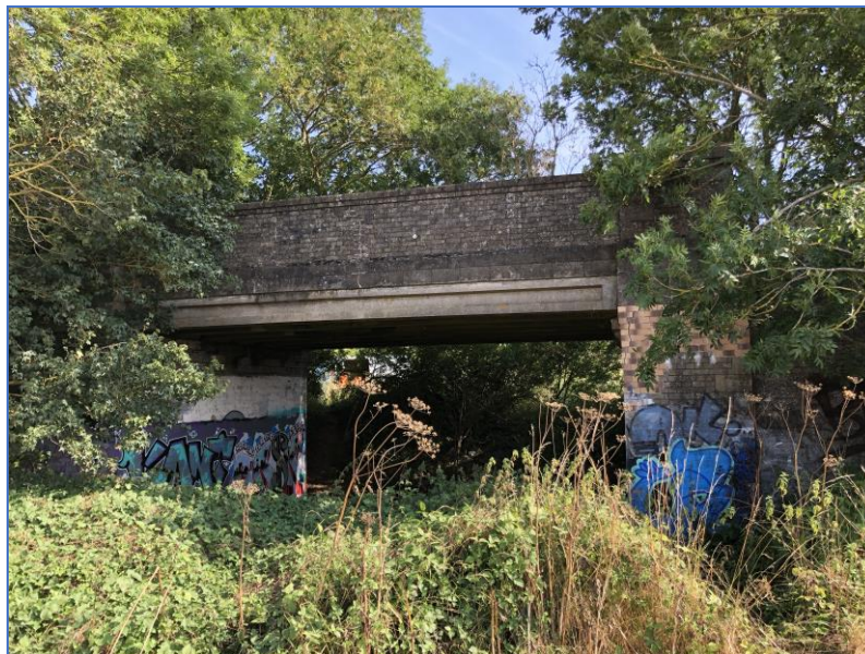
Image 1 - View of south elevation access below structure
