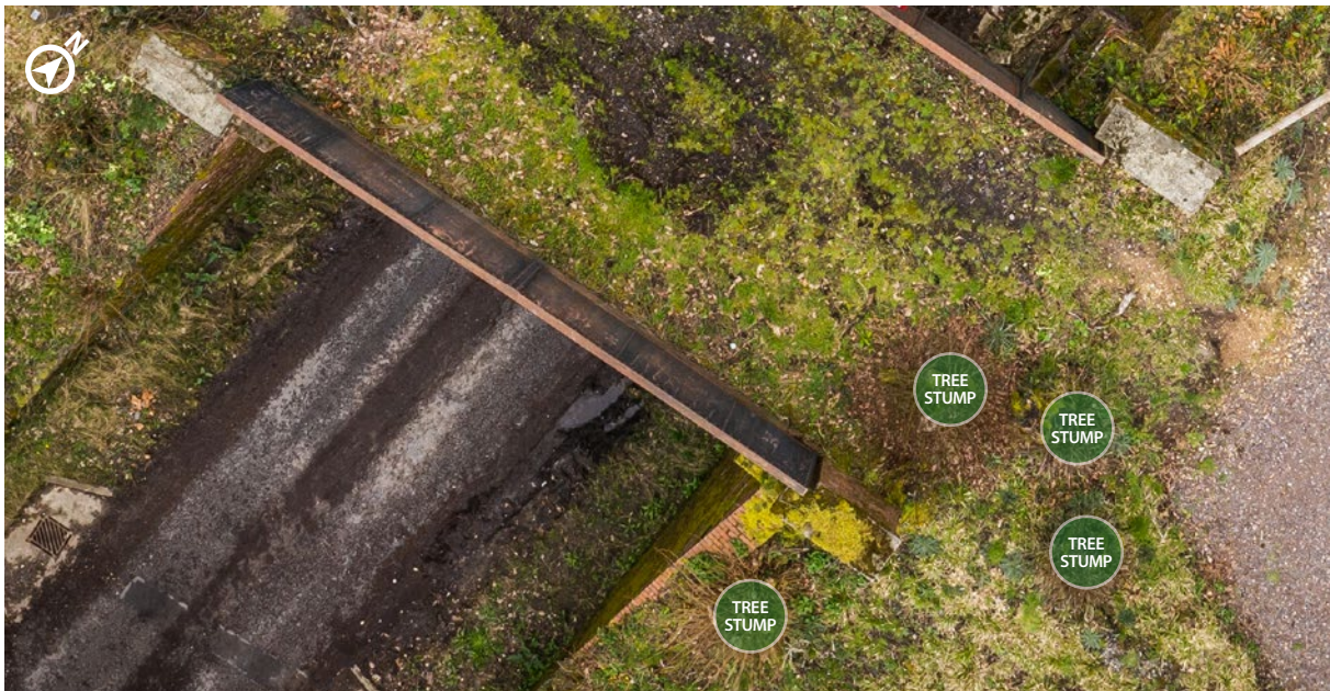
Figure 2: Plan view of felled trees at east abutment and south-east wingwall.
