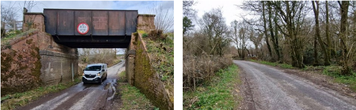
The view north (left) and south (right) from the bottom of the originally intended ramp on the south side of the bridge. The blind bend presents the greatest risk to trailway users.
