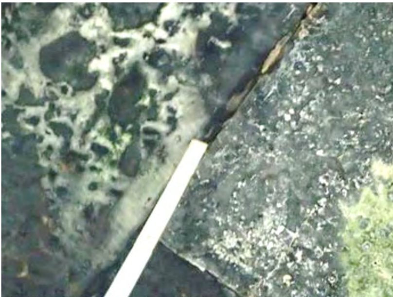
Figure 2.3: Photo 13 from 2020 visual, showing dropped stone with ruler. Ruler sits within chamfer at corners of stones. Where and how was the drop measured on each occasion?
