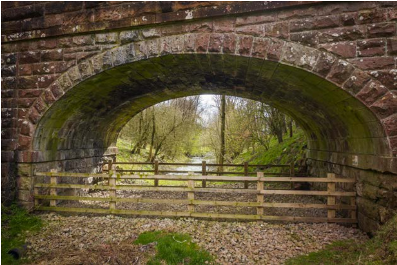
Figure 5.1: A recent photograph showing elevation and soffit.
