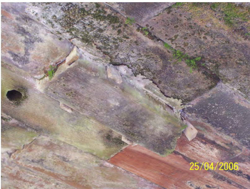
Figure 6.7: A single dropped stone due to mechanical action. Note the clear damage to the surrounding stone, without which the stone could not have dropped this far.
